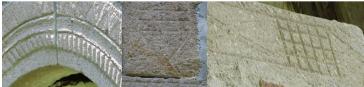
Fig. 11. Motifs carved in stone at the Tower of Salih Kajtazi
