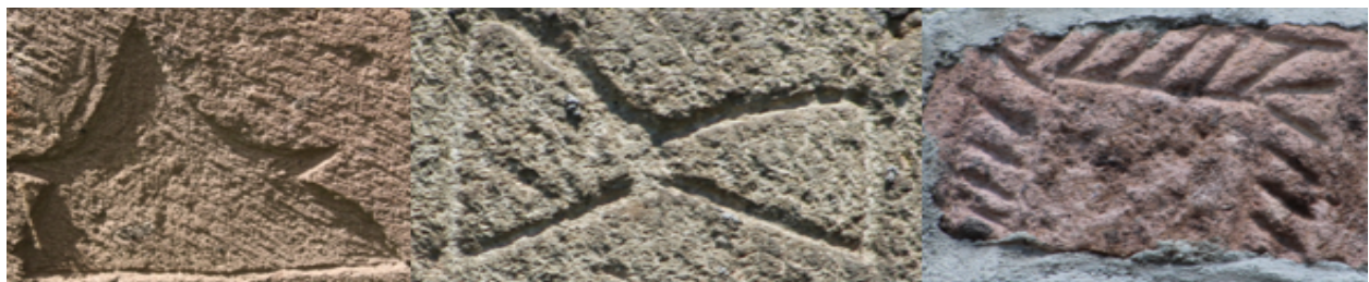
Motifs carved in stone at the Tower of Salih Kajtazi, photos taken by Emin Sallahu and Qazim Namani
